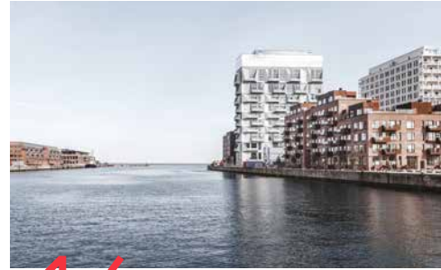
16 Silo in Copenhagen Microtopping®
